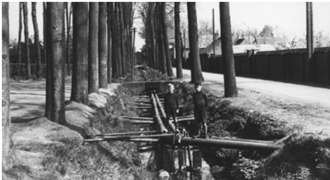
Benzineleiding in De Rips, april 1945.
